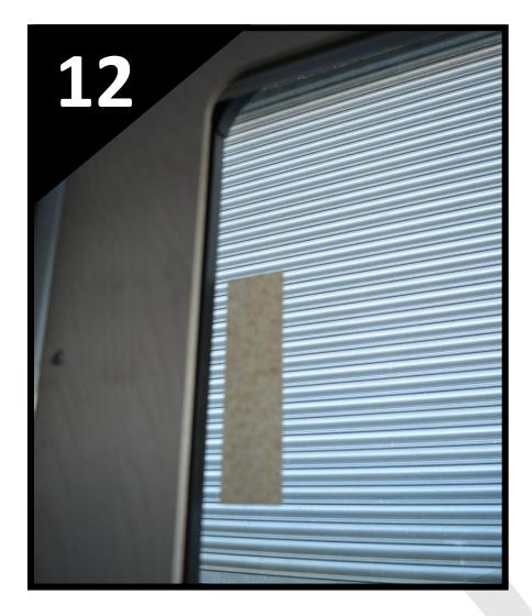
Using some masking tape, tape onto the window roughly where the vertical and horizontal edges of the blind aperture meets the window.
